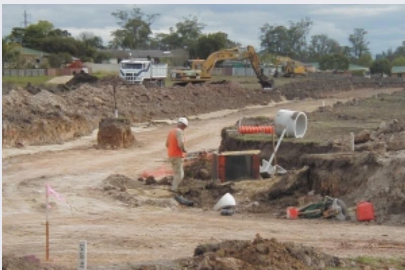
Roadworks and services for Stage 1 are well underway.
